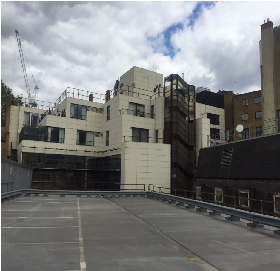
Rear of site from Carrington Street car park
